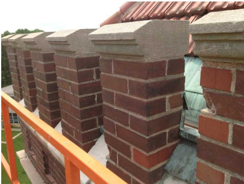
Figure 30. Piers of the east elevation battlement.
