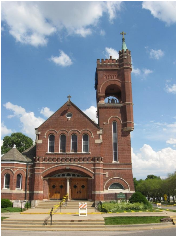
Figure 1. Overall view, west elevation.
