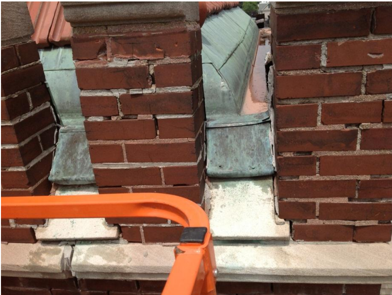
Figure 26. Copper flashing behind battlement, south elevation of bell tower.
