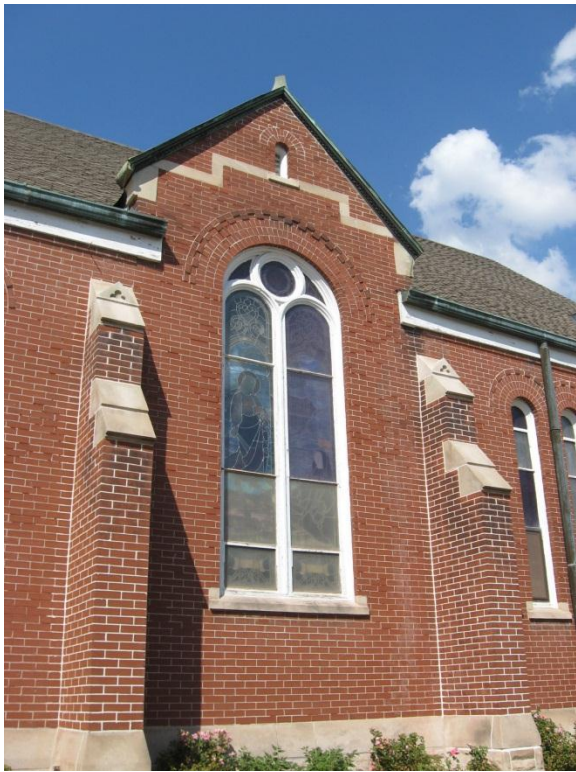
Figure 33. Recently tuck pointed buttresses on south elevation.
