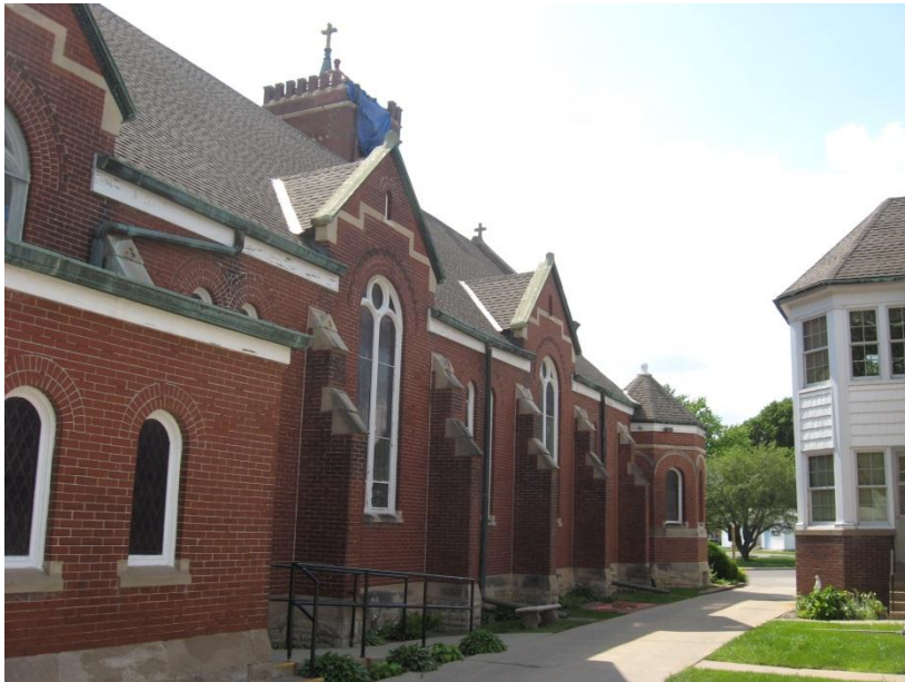
Figure 4. Overall view, north elevation.
