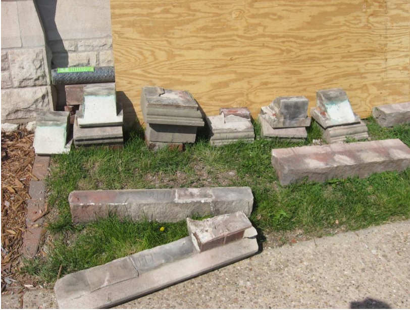
Figure 7. Limestone pieces from north elevation of bell tower stored on ground, south side of church.
