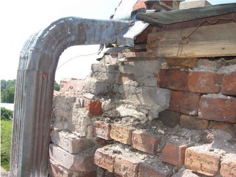
Figure 8. Backup brick masonry removed at northeast corner of bell tower.
