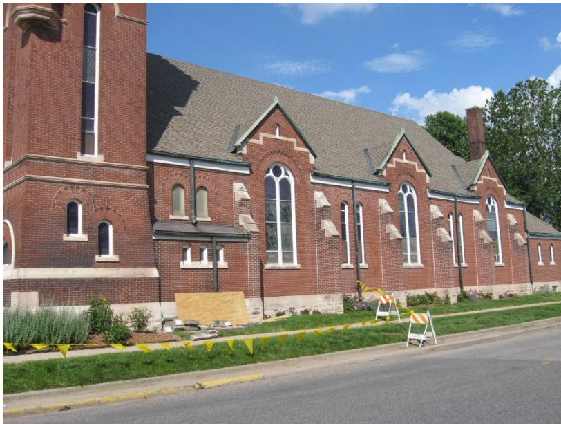
Figure 2. Overall view, south elevation.
