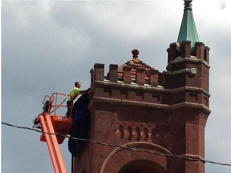
Figure 13. OBC reinstalling tarps at end of WJE/OBC investigation.
