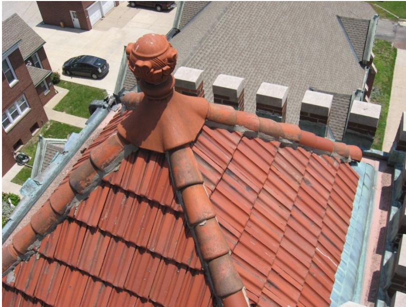
Figure 31. Overall view of bell tower roof.
