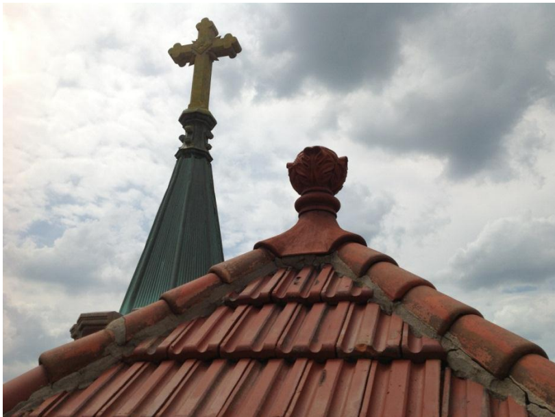
Figure 18. Overall view of steeple, looking over bell tower roof.
