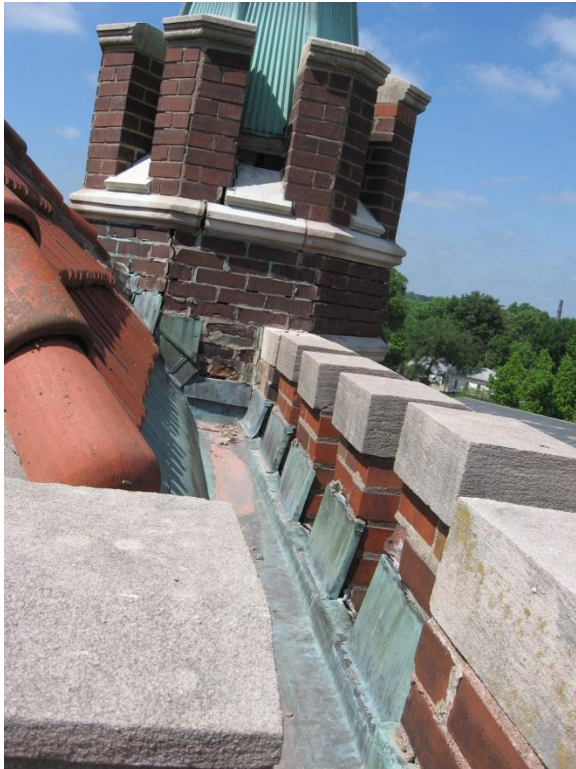
Figure 17. Copper flashing on backside of west elevation battlement.
