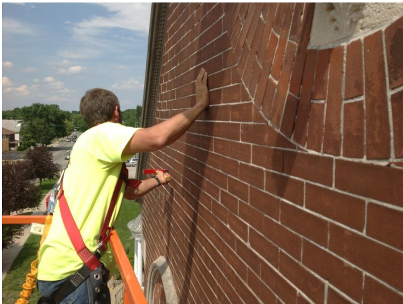
Figure 32. OBC sounding representative portions of west elevation facade above church entry.
